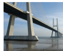
Vasco da Gama Bridge (PT)
