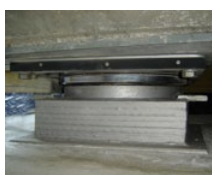
Spherical bearings
