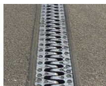
Cantilever finger joint
