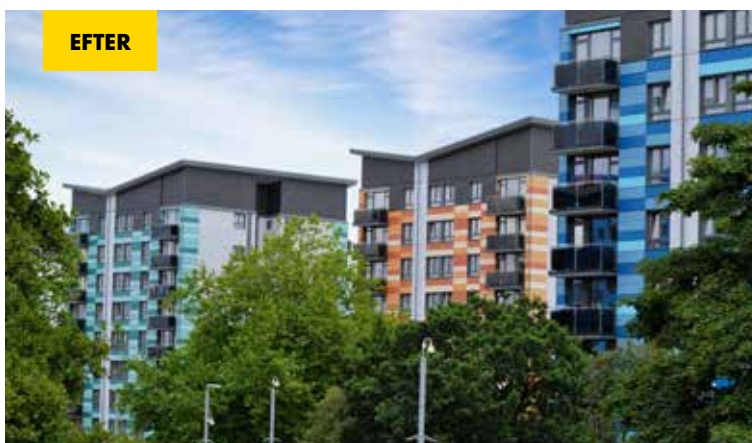
FASADRENOVERING CHARLEMONT FARM ESTATE, UK.
