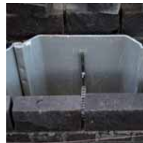
Lateral Brick Wall Support
