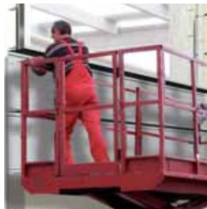
Corrugated Metal Siding & Roofs
