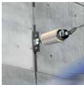
Overhead Electrical Lines
