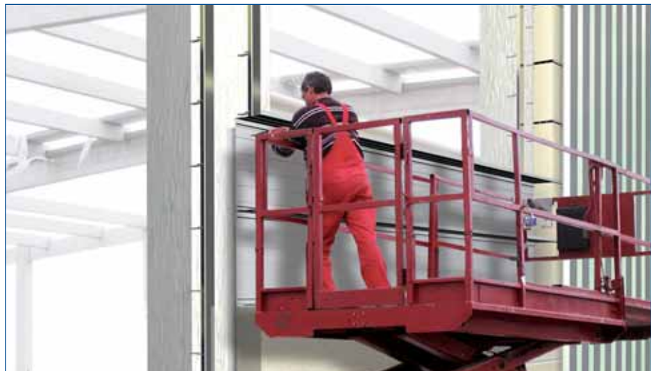
Installation of a Multi-Layer Insulated Corrugated Metal Siding Wall
