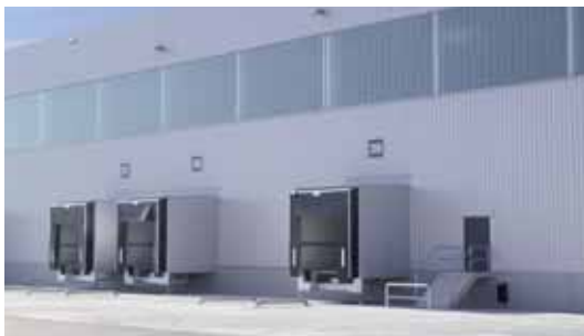
Application to a Wall
