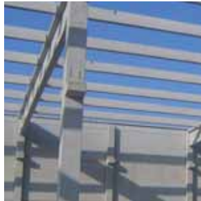
Concrete Precast Elements
