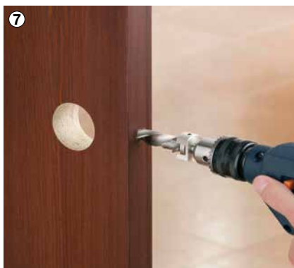
7 Drill hole for latch tube using the HCS® Ø 16.2 mm/22.2 mm stepped drill bit.
