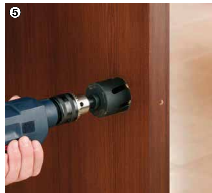
5 Drill 3 mm into door on one side using the Ø 54 mm diameter hole saw.
