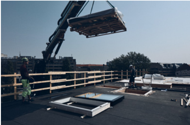
Craning products to the roof
