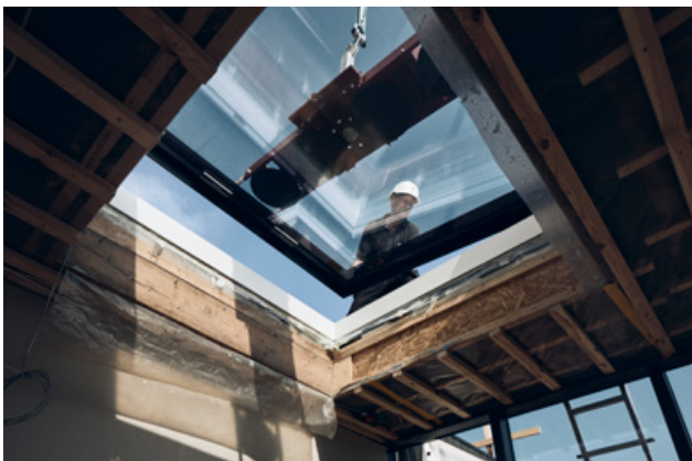
Placing the top unit
