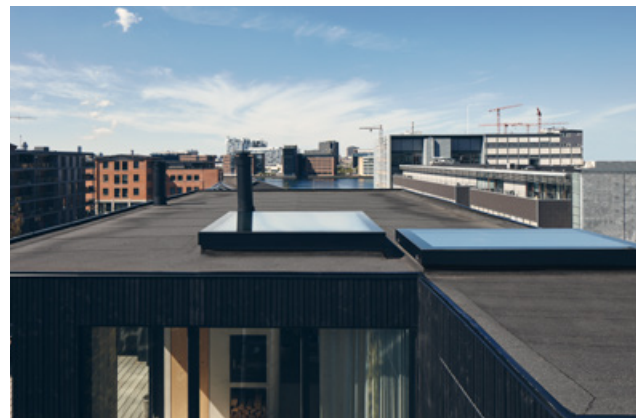
External work finalized
