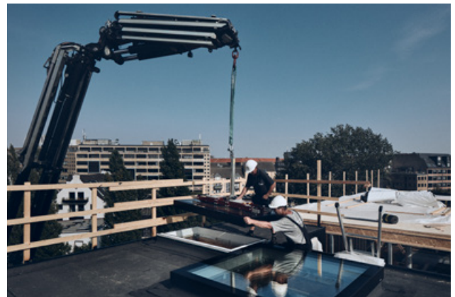
Placing the top unit
