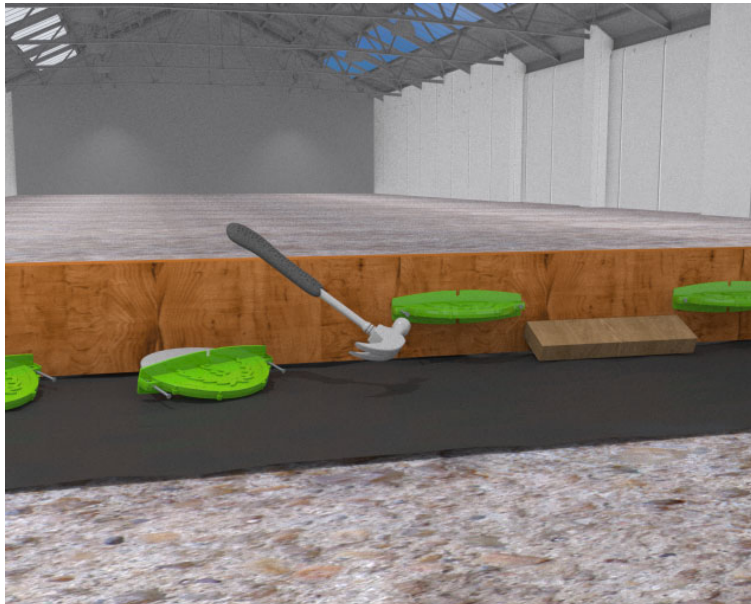
Insert the dowels to the sleeves.
