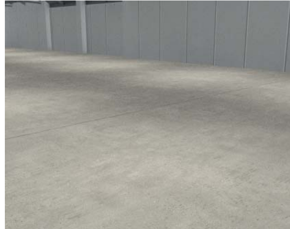
Surface of slab after pouring both sides of screed.
