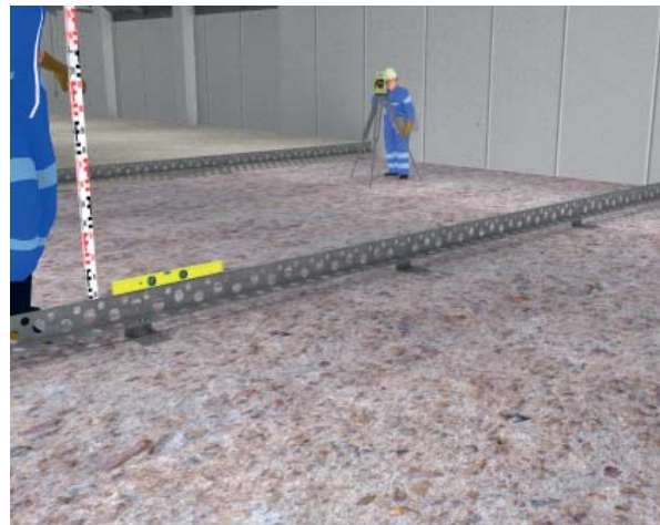
Screws in position after leveling to ensure rails are locked at correct level and position.
