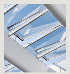
Glazing with electrochrome glass in clear state. Visible light transmission 57%
