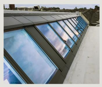
VELUX modular skylights are available with infill panels to accommodate structures, such as a ventilation shaft or an existing wall construction. Infill panels can also be used on the south-facing side of a Ridgelight to imitate a shed roof structure.
