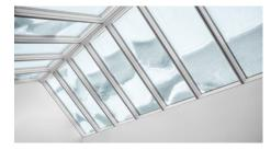
Low-energy glazing in combination with low-conductive profiles create an effective shield against all kinds of cold weather.
