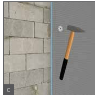
C Insert wedi Tools metal dowels in the holes and hammer in after the mortar has fully dried.
