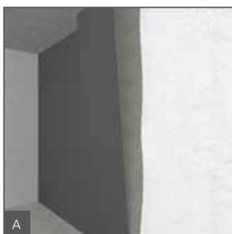
A Attach the wedi Vapor building boards across the full surface with tile adhesive.
